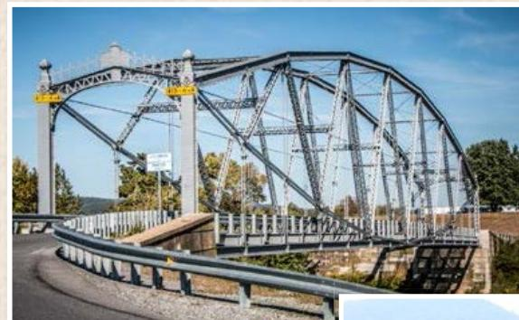
The nearly 288-foot long Pine Creek Lenticular Truss Bridge near Jersey Shore is one of only about 50 truss bridges still standing in the United States.
