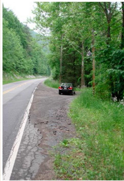
Provide safe turn-outs. Turn-outs can be simple (like this) or enhanced with interpretive signage or viewing platforms.
