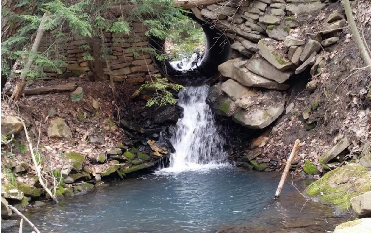
Figure 47 - Collapsing Culvert Rock Wall in Clearfield County
