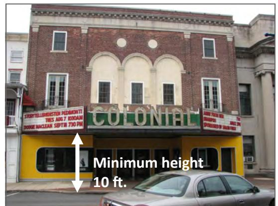
*A minimum vertical clearance of 10 feet is required between the bottom of the marquee sign and the sidewalk.*
