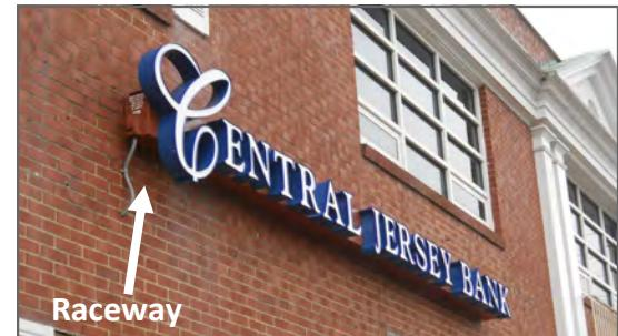
*The letters of an internally-illuminated wall sign are usually applied to a "raceway," which houses the electrical components, rather than directly to the wall itself. However, typically the "raceway" is interpreted to be a part of the sign.*
