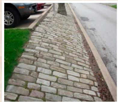
Use infiltration features for roadside drainage system
