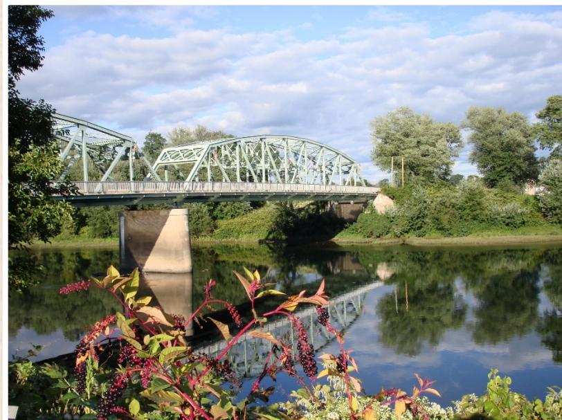
The two-span Jersey Shore Bridge, rehabilitated in 2000, is one of the last remaining truss bridges on the West Branch Susquehanna River.
